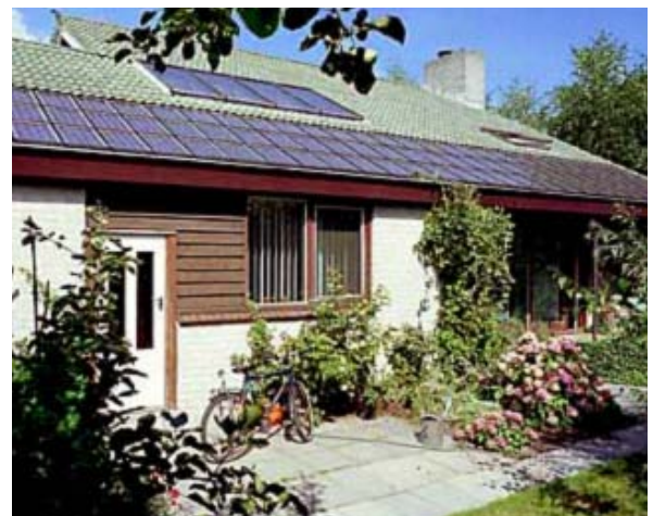
An average North Carolina homeowner can now have a solar electricity system installed for a net cost ranging from $8,200 to $20,000 or more, depending on how much electricity the homeowner wants to generate.
